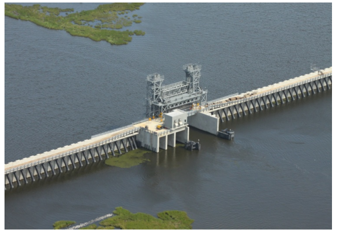
Vertical Lift Gate at Bayou Bienvenue
