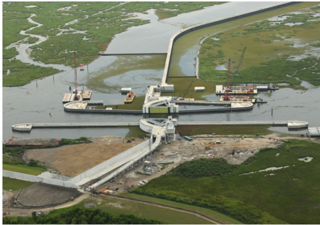
Barge Gate and Sector Gate at the Gulf Intracoastal Waterway
