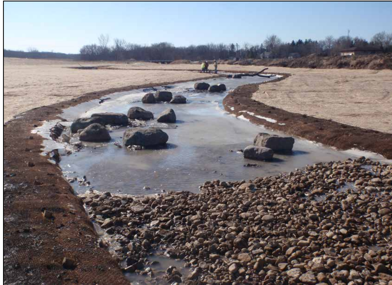
The Pike River Ecosystem Restoration Project in Wisconsin moved more than 600,000 cubic yards of material to restore and enhance a low-flow channel. In-stream improvements made to the Pike River help provide diverse habitats in the riverbed. (Courtesy photo)
