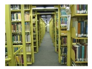
The stack tiers are self-supporting and as is typical in such a design don't correspond to the regular floors of the building. The stacks include some individual study spaces, but are very inflexible.
