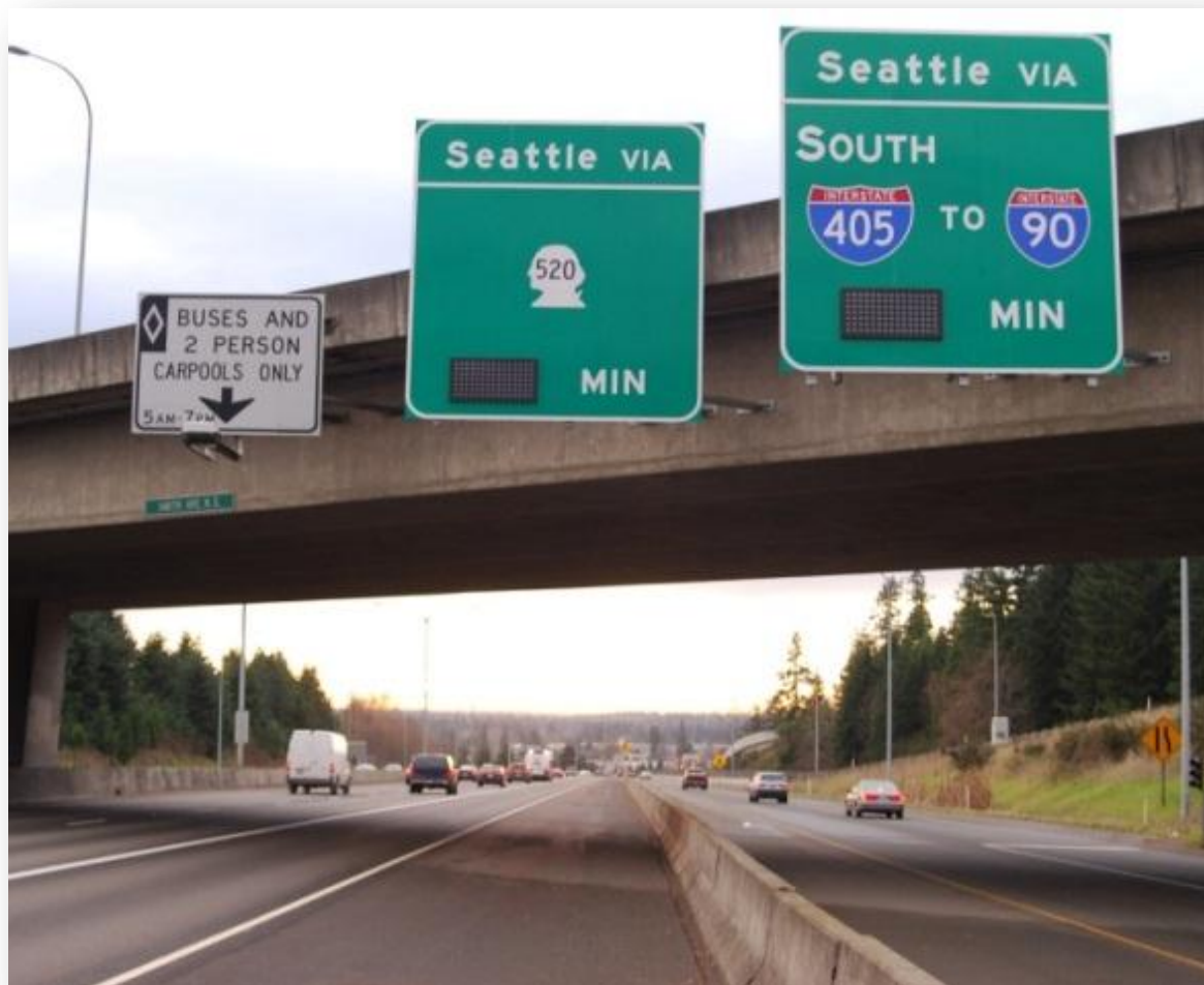
Figure 2. Travel time signs, Seattle, Washington (Source: WSDOT).
