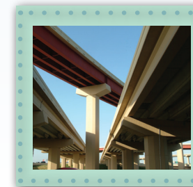
Overpass $6.8 million per lane mile
