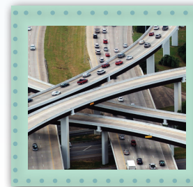
Freeway Interchange $325 million
