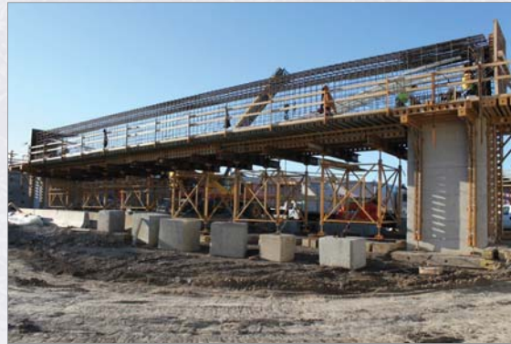
Constructing bridge substructure for southbound TEXpress lane entrance from Basswood Blvd.
