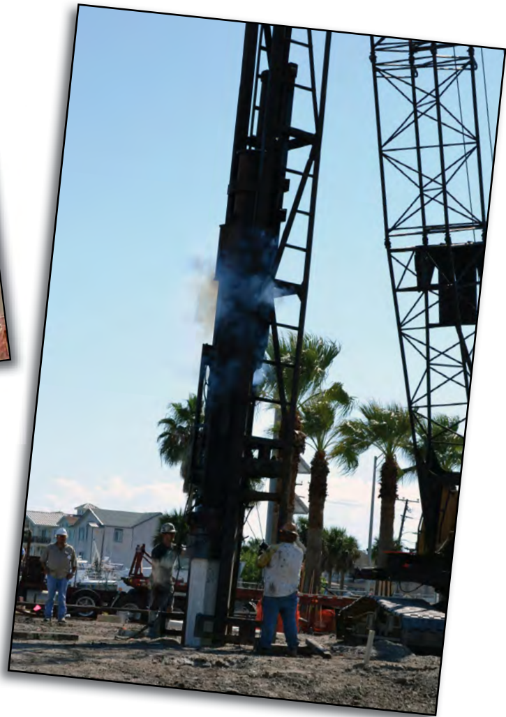
Pictured above brick masons begin building the walls for the new Ferry Operations Building in February. At right, the first piling is driven into the ground prior to the laying of the foundation.
