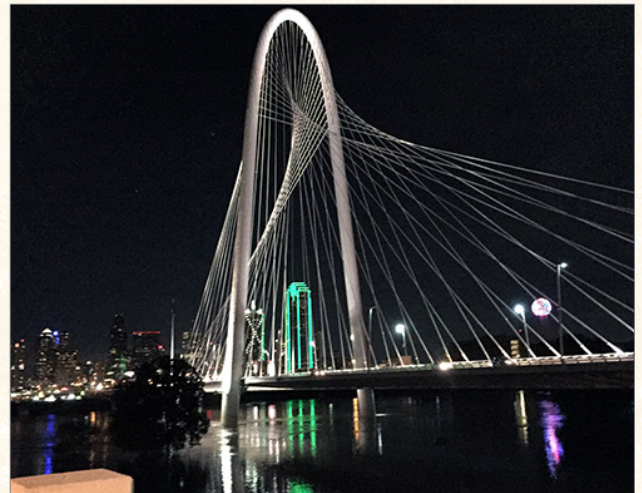
Rising water in the Trinity River creeps close to the bottom of the Margaret Hunt Hill Bridge.
