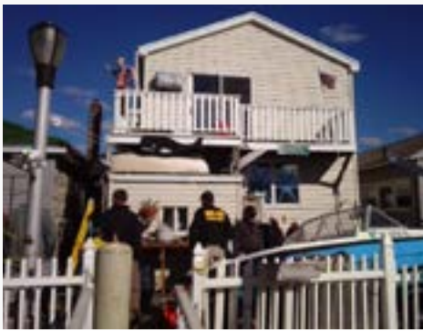
Special Agents assessed the damage and hazardous situations around assigned sites.
