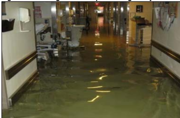
Figure 2: Flooding in One Hospital During Sandy
