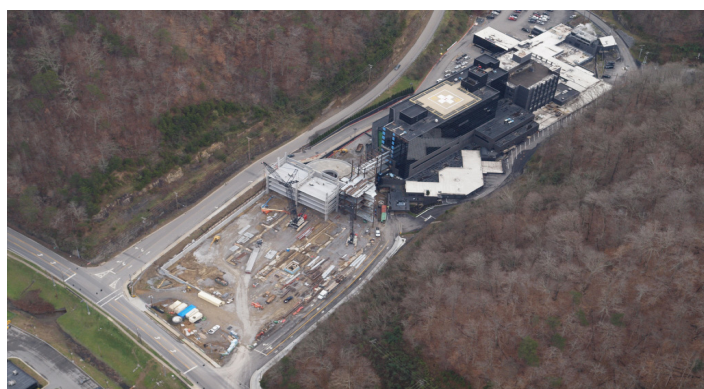
Pikeville Medical Center added a new medical office building and garage.
