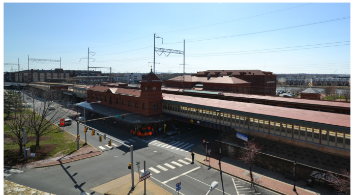
Amtrak's renovated station in Wilmington, Delaware has won a Brunel Award for design.
