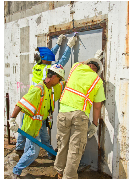
Workers seal one of the reactor doors.
