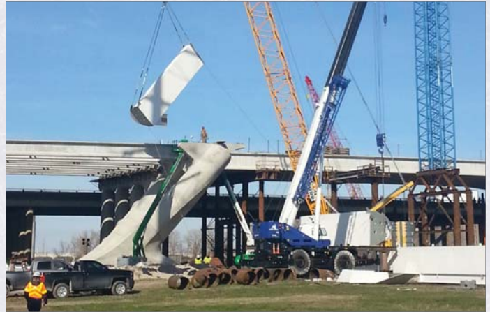
The first steel sections of the Margaret McDermott Bridge on I-30 over the Trinity River arrived in mid-November and crews installed the first section of the eastbound arch on January 7, 2015.
