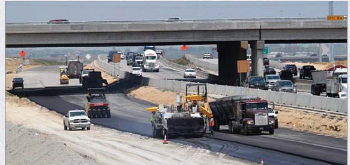
Constructing the southbound general purpose mainlanes at Basswood Blvd.
