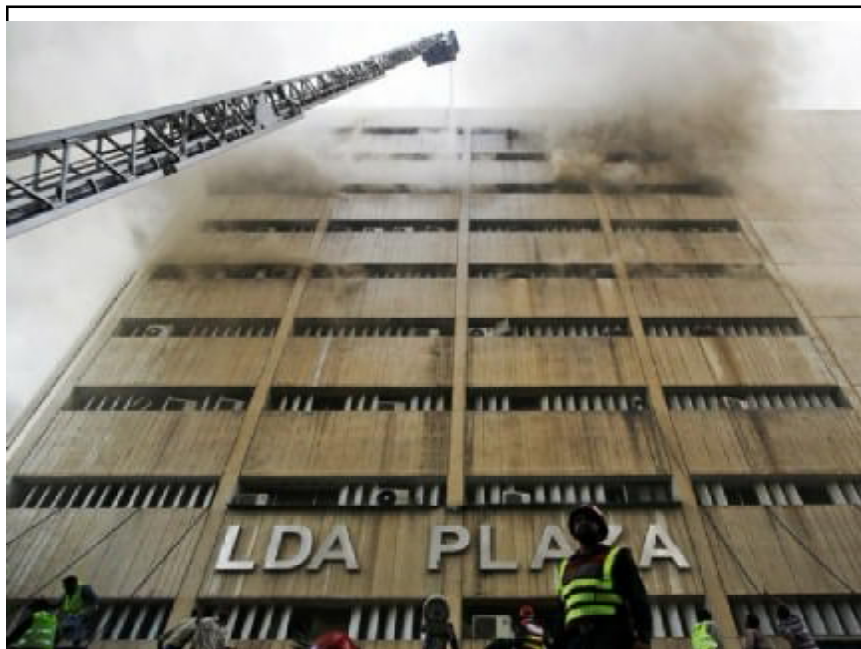
The LDA Plaza fire exposed safety measures at the office of the authority responsible for ensuring compliance with safety and other by-laws.
