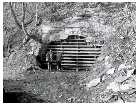
Staff inspecting bat gate closure installed at Brooklyn Mine, New River Gorge National River, West Virginia.
