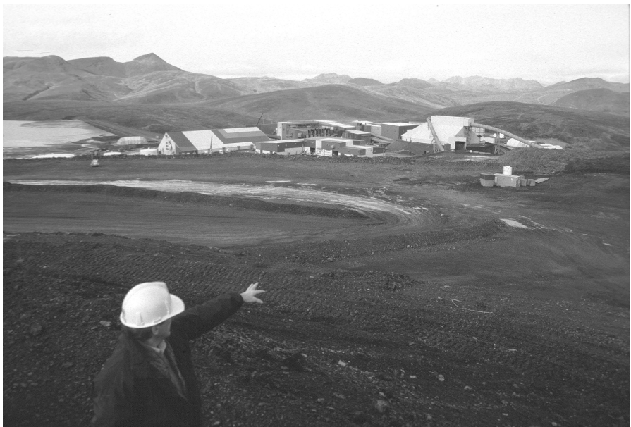
Red Dog Mill and Employee Residence - Jim Kulas, Environmental Manager at the Red Dog Mine, explains water quality monitoring at the lead/zinc floatation mill.
