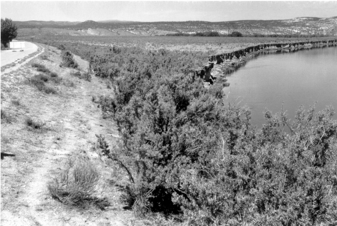
View looking downstream (west) of the eroding left bank of the Yampa River and the Deerlodge Park access road on June 29, 2000.
