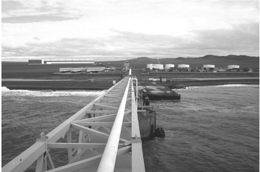
Delong Mountain Port Facility - Over 1.4 million tons of lead and zinc concentrates, 36,000 tons of fuel, and 17,000 tons of chemical reagents, food, equipment and supplies pass through the port facility (and the Monument) each year.
