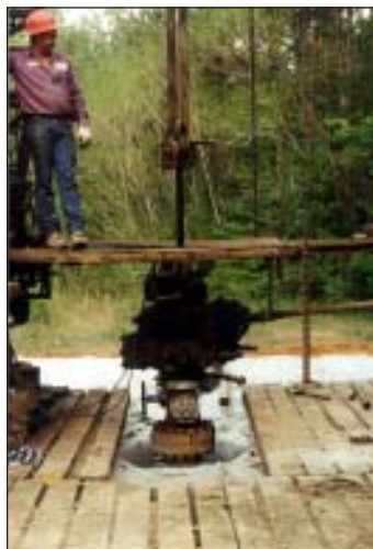
An oil and gas operator plugs and abandons a gas well in Big Thicket National Preserve. Photo by Pat O'Dell.
