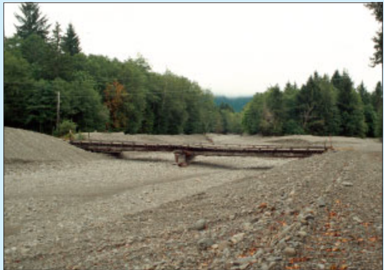
Park Maintenance extracts gravel from Finley Creek Bridge at Olympic National Park to protect the bridge and maintain flows. Photo by Mark Ziegenbein.
