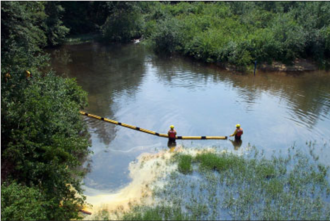
In an effort to contain the oil spill, responders to the oilwell blowout in Obed Wild and Scenic River deploy a boom. NPS photo.
