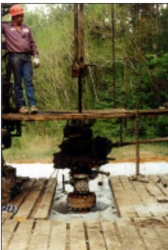
An oil and gas operator plugs and abandons a gas well in Big Thicket National Preserve. Photo by Pat O'Dell.
