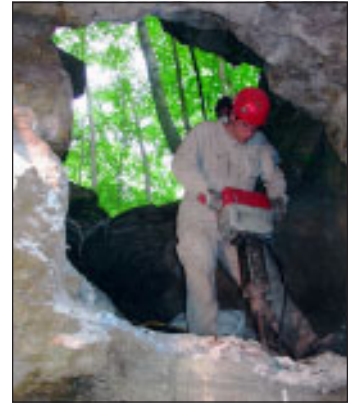
Through the Geological Society of America GeoCorps Program, Dan Clark was a Geoscientist-in-the-Parks at Mammoth Cave National Park. His work on the Lesser Cave Inventory included measuring cave entrances, writing descriptions, taking digital photographs, and recording GPS locations. Dan's work also included cave restoration, such as the removal of a concrete wall to restore natural air flow to the cave. Photo by park staff.
