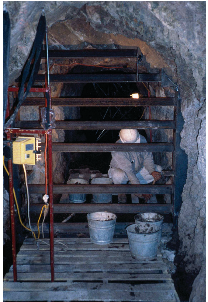
A bat gate installation at Saguaro National Park.
