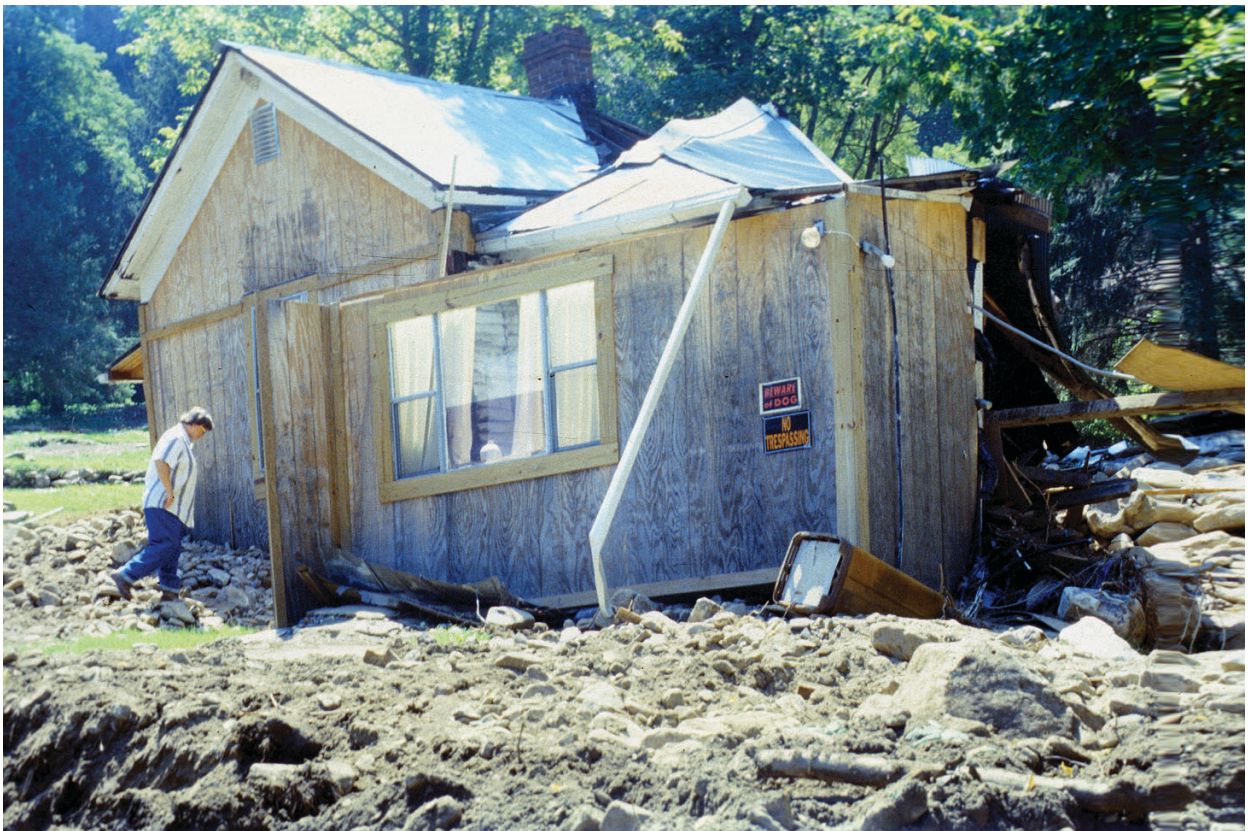
Local resident of Thayer, WV, next to remains of her house destroyed by a boulder debris flow.
