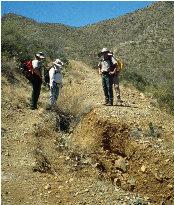
Roads divert surface flow and cause accelerated erosion, even in arid environments such as Saguaro NP.
