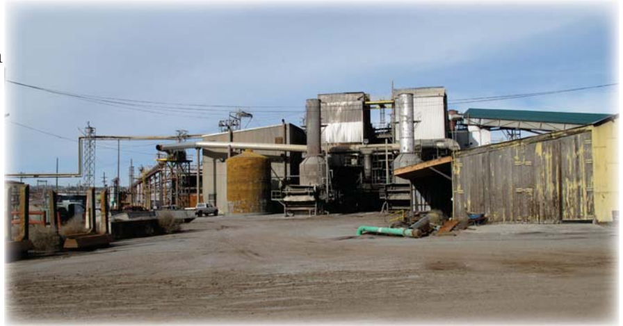
CIPV Biomass Generation Facility. File Photo.
