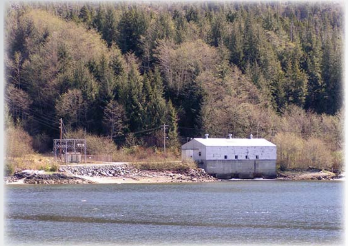
Figure 2: Purple Lake Hydroelectric Plant
