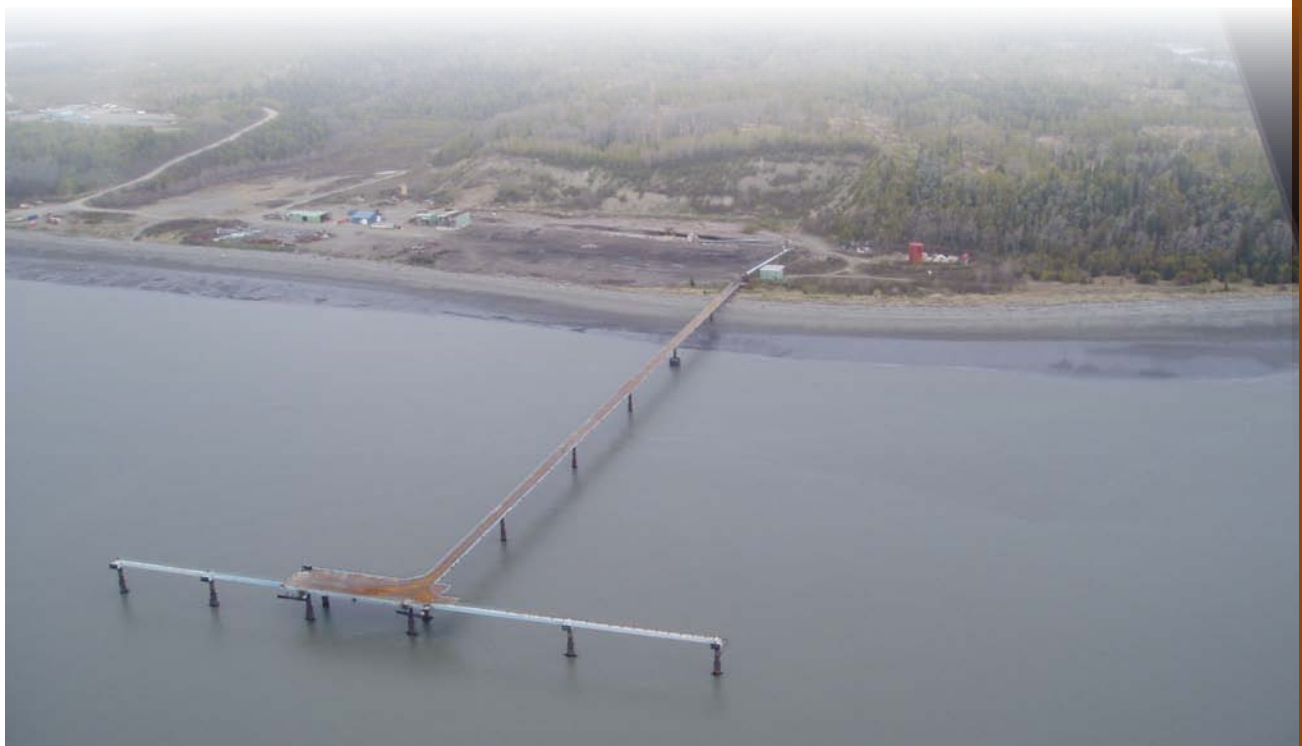
Figure 3: North Foreland Facility (NFF)
