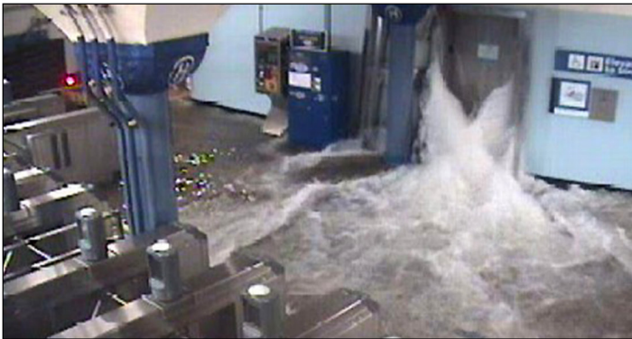
Flood waters pouring into the Hoboken Station on the Port Authority Trans-Hudson (PATH) System
