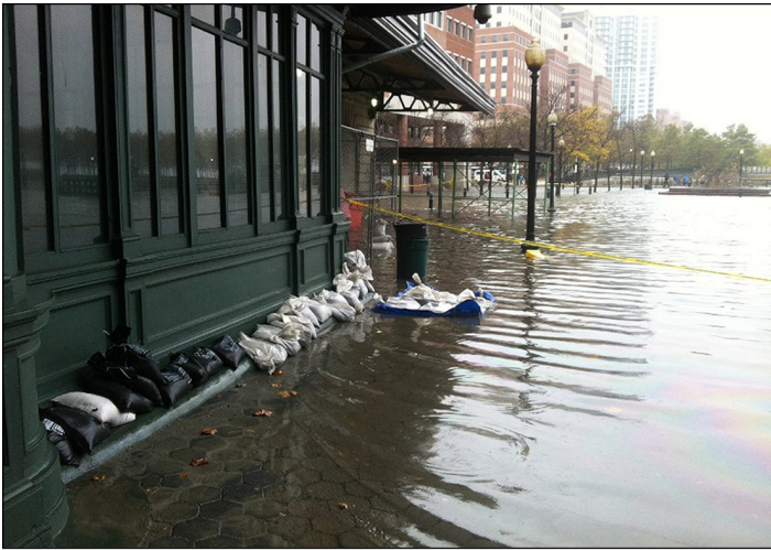
Sandbags at the entrances of Port Authority Trans-Hudson rail transit station in Hoboken, N.J.
