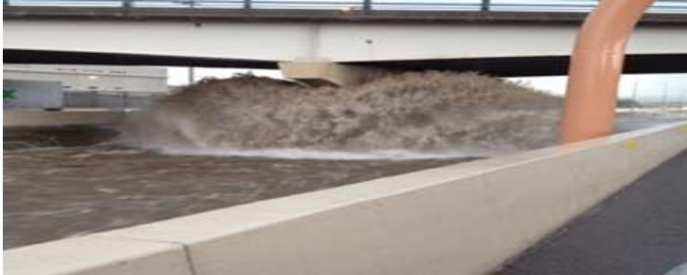
Figure 1. Flooding in DR-4148
