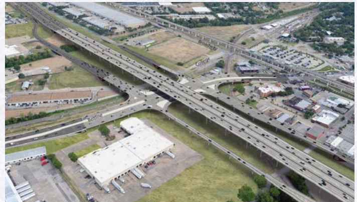
Photo rendering of the future Belt Line/I-35E interchange now under construction looking north.
