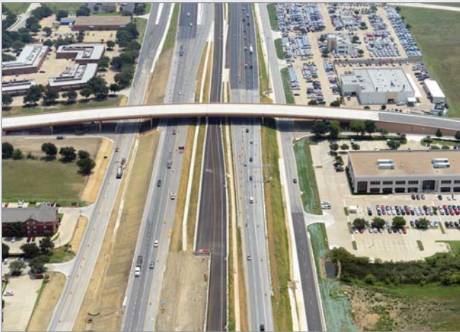
Pictured above: The new Riverside Drive bridge over I-820
