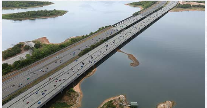
Photo rendering of the new southbound Lewisville Lake Bridge.
