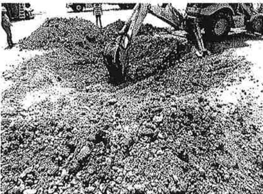
Photo #5 View of the pit excavation.
