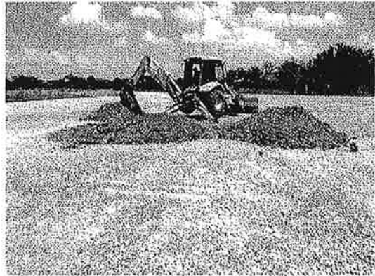
Photo #4 View of the pit excavation.
