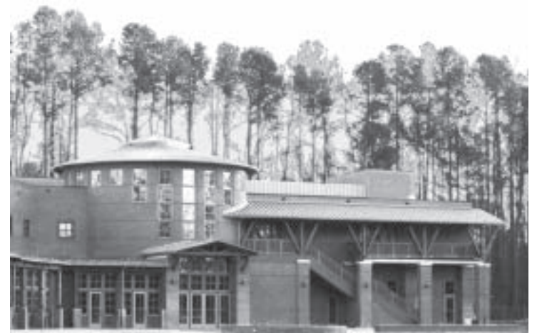
Jamestown Settlement's new theater and special exhibition wing neared completion in 2003.
