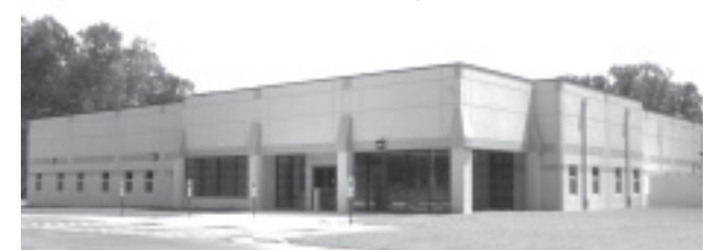
Central support complex
