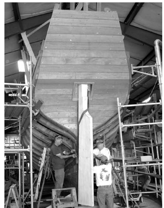
Shipwrights temporarily install the new Discovery 's rudder to prepare patterns for rudder hardware.
