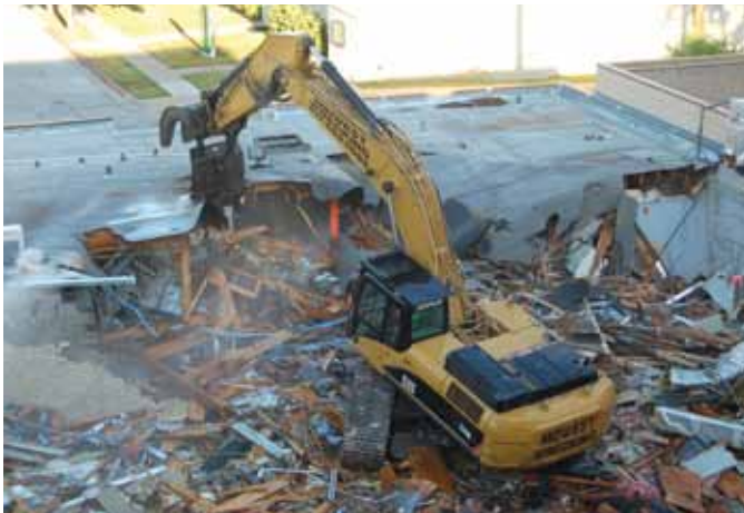
Demolition in progress as viewed from the library
