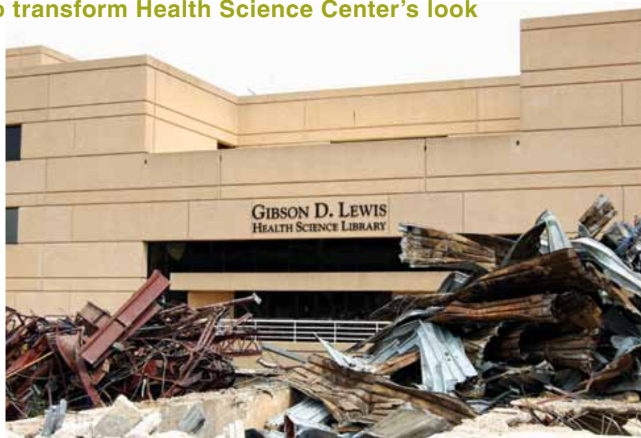
Building debris sorted and ready for recycling
