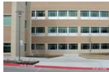
Chemistry Building - ribbon windows
