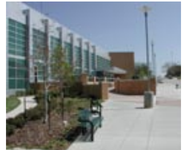
Student Recreation - south facing curtain wall and metal panels.
