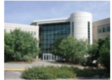
Environmental Education - south facing curtain wall
