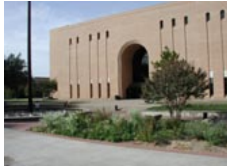
Willis Library - east facade & entry
