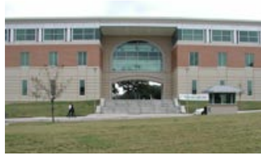
Gateway Center - archway
