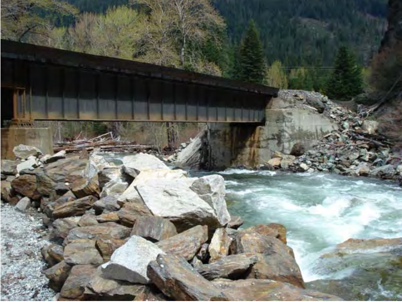
Figure 9. Downstream view to the north at riprap placed along USFS road and White Pine Railroad Bridge abutment near assessment area boundary (RM 14). (Reclamation photograph by R. McAfee, May 2, 2007).
