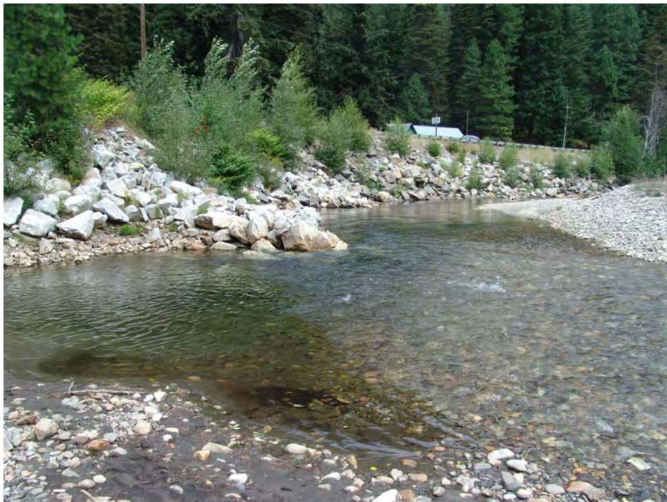
Figure 32. View is to the northeast looking downstream, showing riprap with two rock spurs into channel at RM 13.3. (Reclamation photograph by D. Bennett, August 7, 2007).
