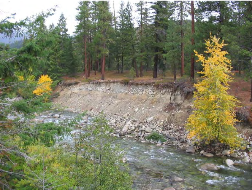
Figure 45. Looking at eroding glacial bank on left side of river in section where highway has cut off the historical meander bend near RM 6.6. (Reclamation photograph by D. Callahan, October 9, 2007).
