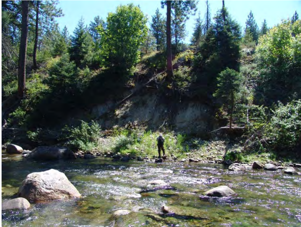
Photograph No.34. View is to the east showing bank profile site on right bank. Nason Creek - Wenatchee Subbasin, Washington. (Reclamation photograph by D. Bennett, August 9, 2007).
