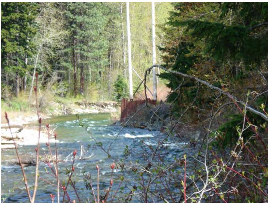
Figure 30. Downstream view to the east of sheet pilings that protect the power pole near RM 13.5
