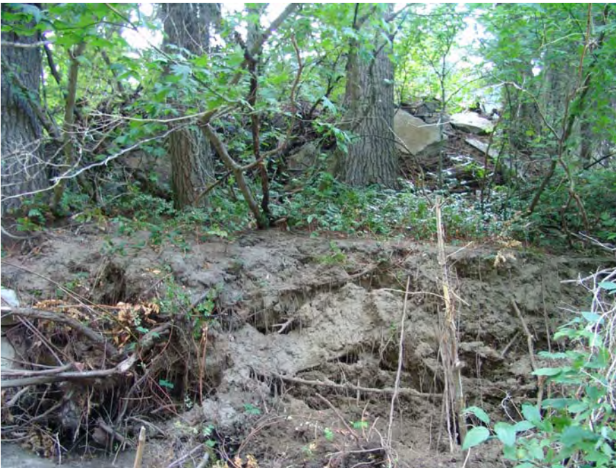
Figure 24. View is to the south looking at the right bank showing original ground level with fill material on top at river bank adjacent to Merritt. (Reclamation photograph by D. Bennett, August 8, 2007).
