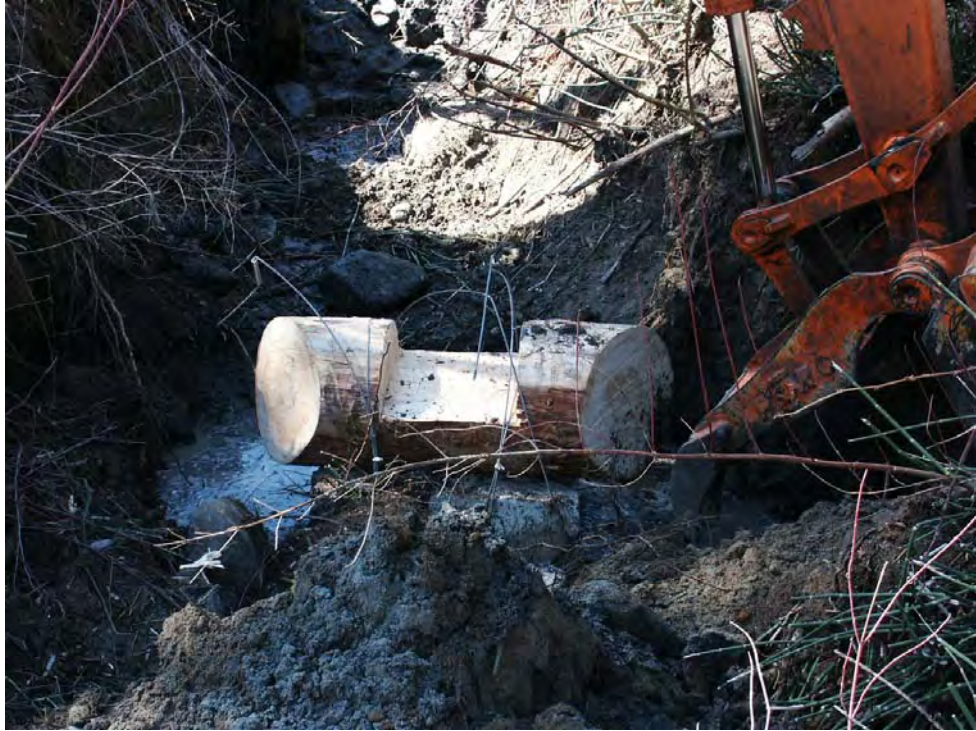
Photo A-7. Weir No. 6 (downstream-most) was placed first.
