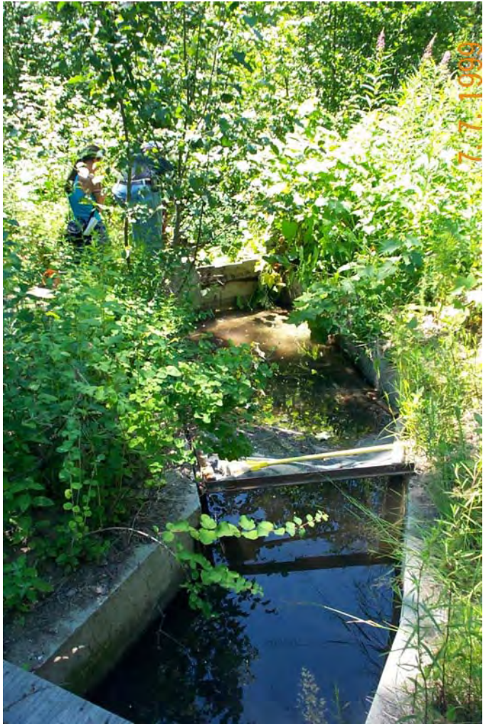
Photo A-2. Mill Creek Diversion ditch, looking upstream, circa July 1999. (photo by Chelan County Conservation District)
