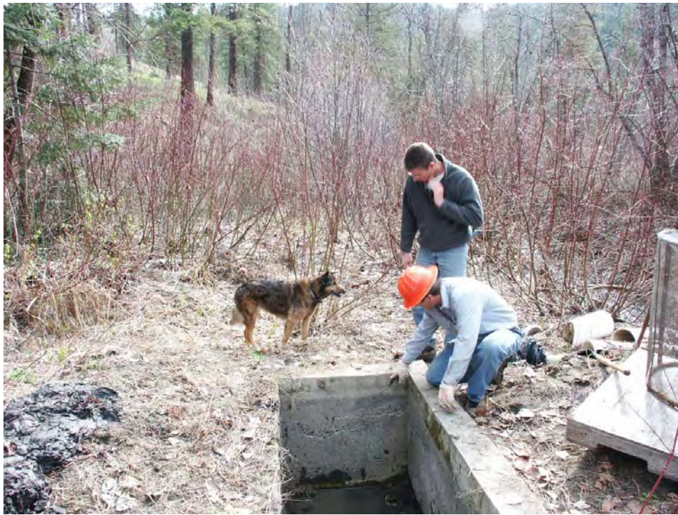
Photo A-3. Existing Mill Creek Diversion structure prior to construction.
