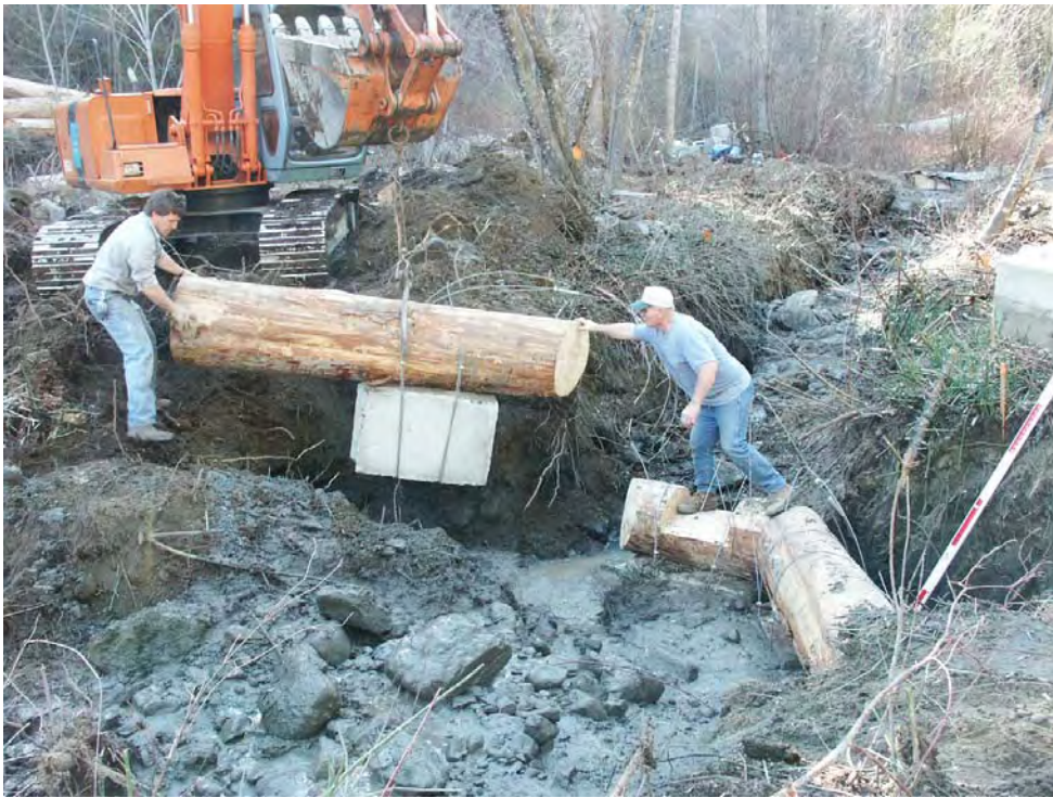
Photo A-9. Maneuvering right-side arm for Weir No. 6 into place.
