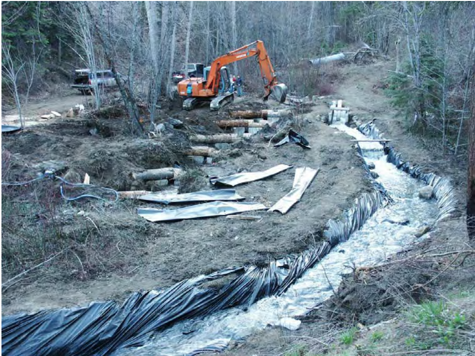
Photo A-12. Panoramic shot (looking upstream) at temporary bypass and weirs.
