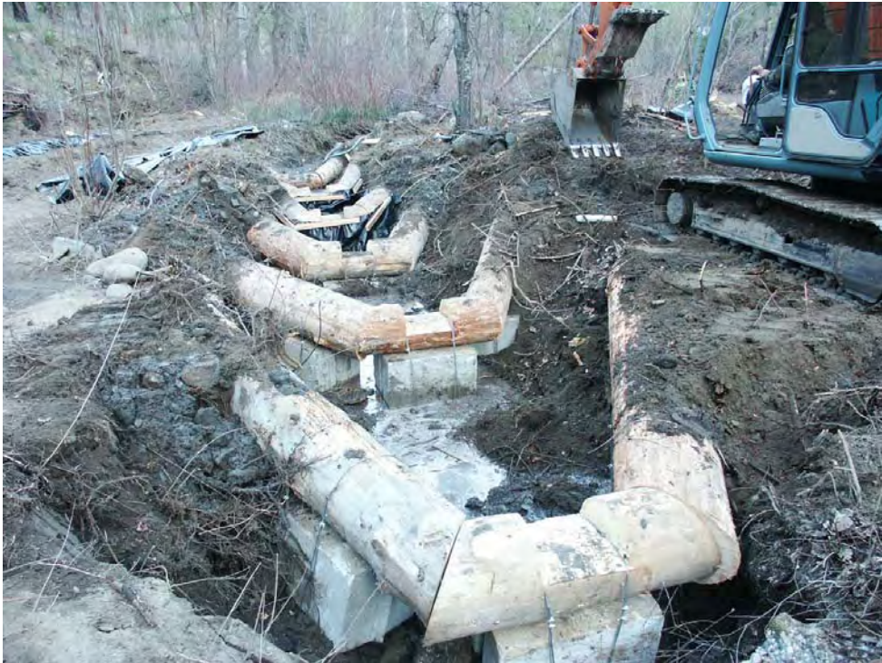
Photo A-11. Backfilling between weir arms, looking downstream.
