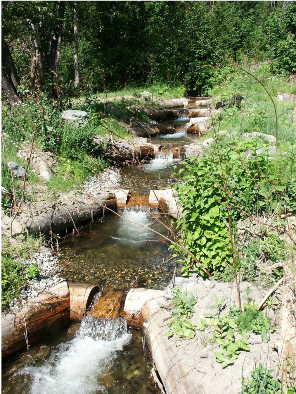
Photo A-19. The new Mill Creek Diversion weirs, six months after revegetation; note gravels visible in ponds.
