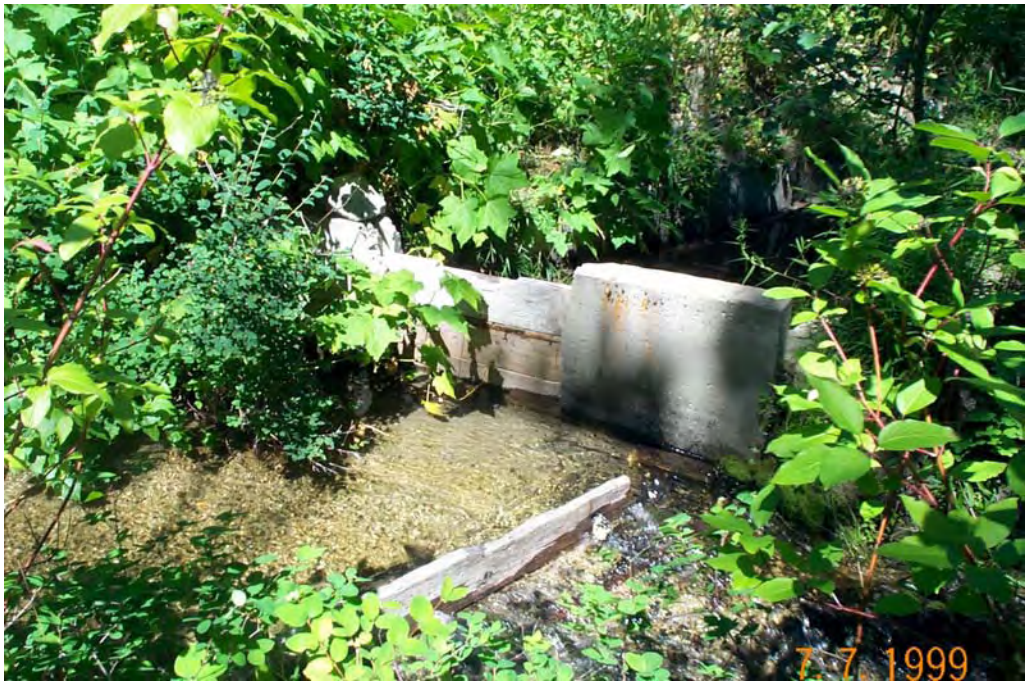
Photo A-1. Mill Creek Diversion, July 1999. (photo by Chelan County Conservation District)
