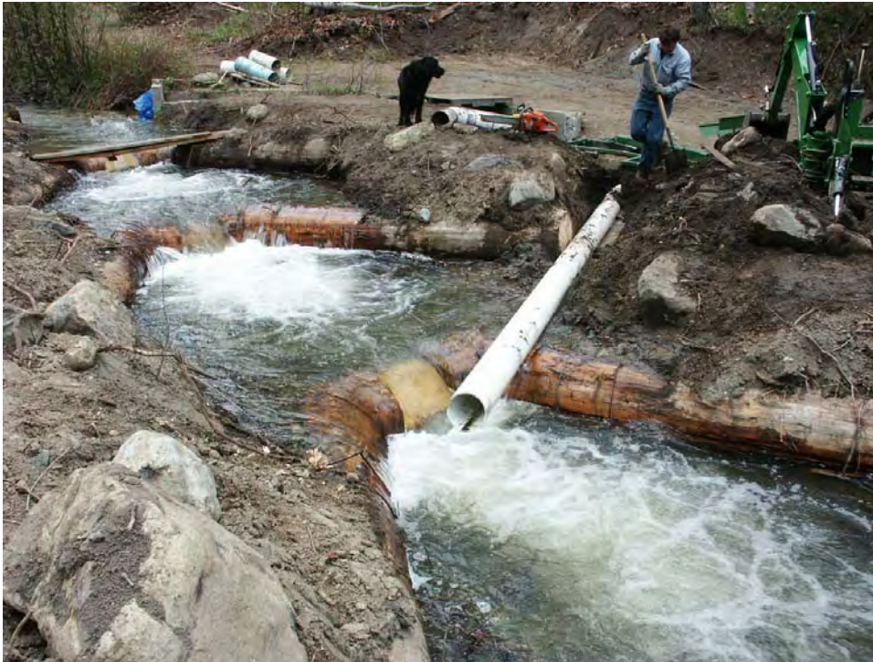
Photo A-17. Final bypass pipe alignment.
