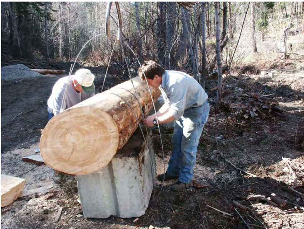
Photo A-8. Fastening an angle-cut arm to an "ecology block" pier.
