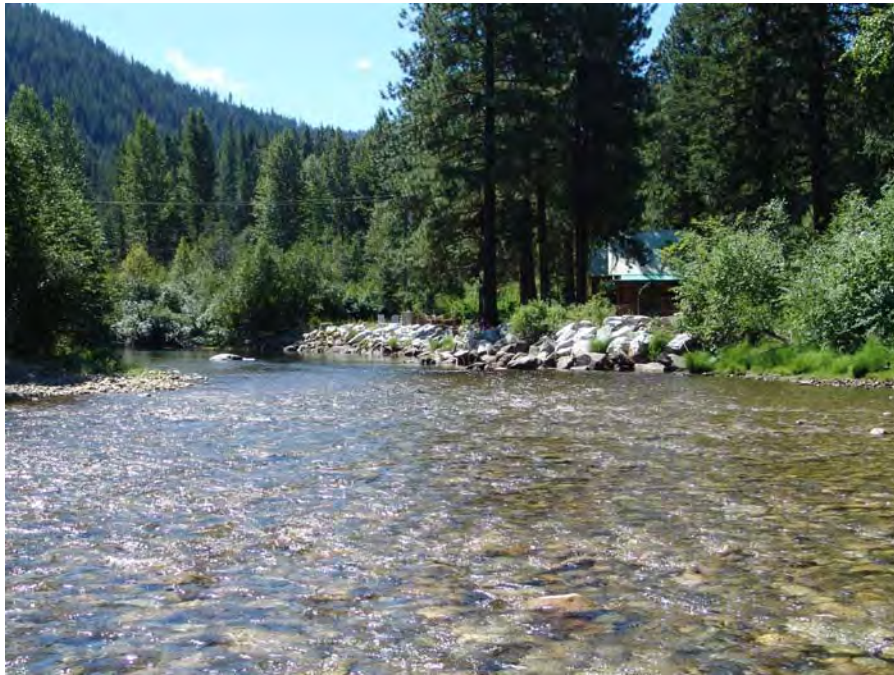
Photograph No. 20. View is to the south looking downstream showing a channel unit sequence of rifle to run and riprap protection along right bank. Kahler Reach; Subreach IZ-1, Nason Creek - Wenatchee Subbasin, Washington. Bureau of Reclamation Photograph by D. Bennett 8/9/07.
