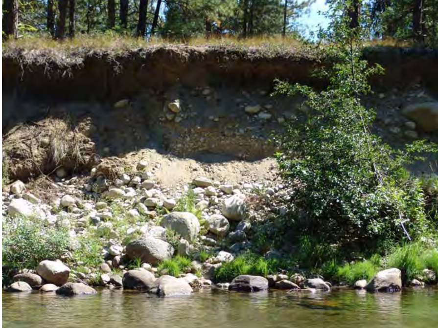
Photograph No. 8. View is to the east showing local erosion of the terrace along the right bank. Composition is a mixture of sand with gravels cobbles and boulders. Kahler Reach; Subreach IZ-2, Nason Creek - Wenatchee Subbasin, Washington. Bureau of Reclamation Photograph by D. Bennett 8/9/07.
