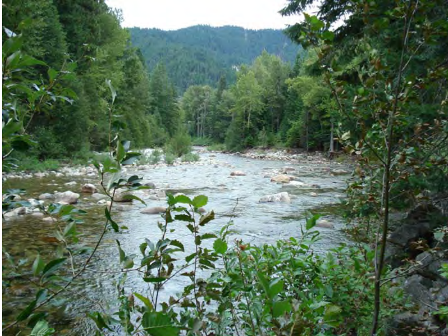
Photograph No. 11. View from the right bank looking downstream to the south east at in-channel boulders and riprap along the right bank. Kahler Reach; Subreach IZ-4, Nason Creek - Wenatchee Subbasin, Washington. Bureau of Reclamation Photograph by R. M o Affee, August 12, 2007.
