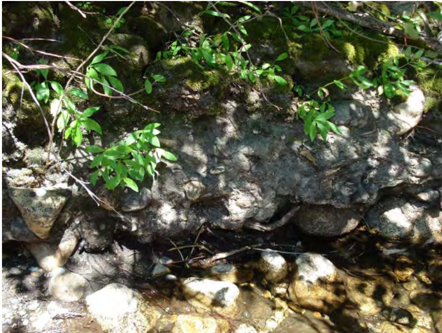
Photograph No. 21. View to the north showing minor undercutting of the lowest surface in a succession of terraces along the left bank of the river. Kahler Reach; Subreach IZ-2, Nason Creek - Wenatchee Subbasin, Washington. Bureau of Reclamation Photograph by R. M o Affee, August 10, 2007.
