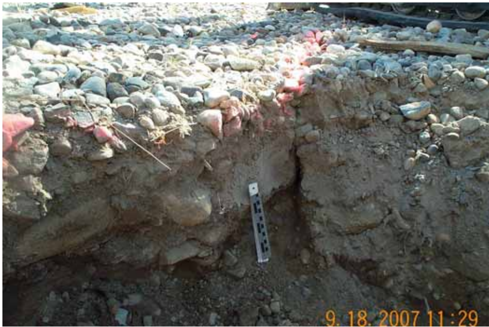
Photograph No. 12. View is to south looking at an excavated extension crack that generally dips to the east toward the river exposed in test pit TP-07-1. Fulton Dam, Methow Subbasin, Washington – Bureau of Reclamation Photograph by E. Lyon, September 18, 2007.
