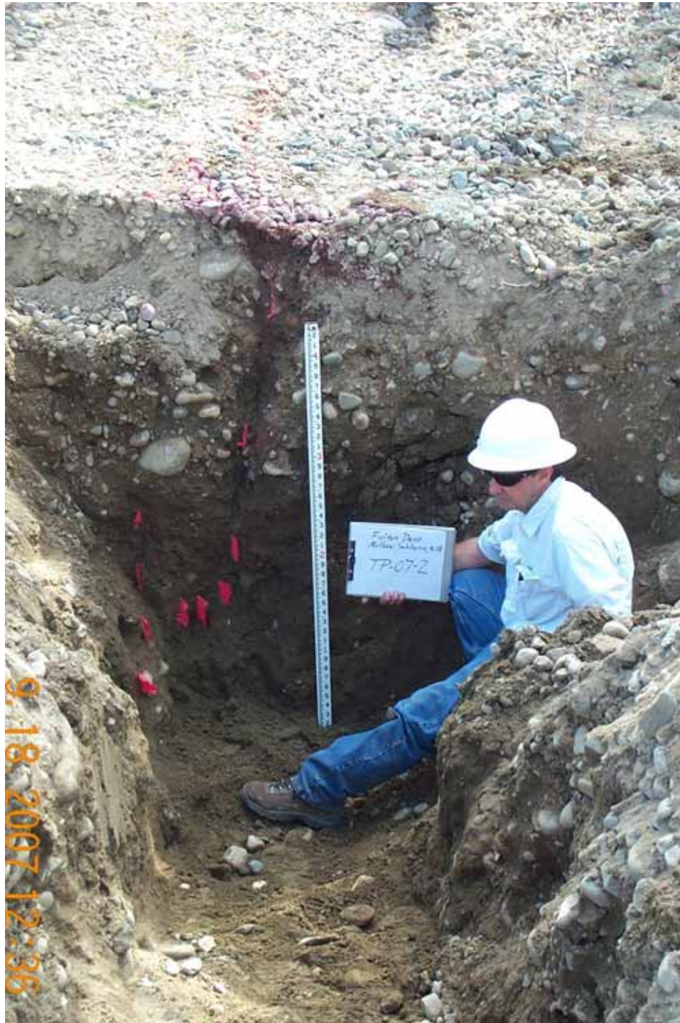
Photograph No. 6. View is to the south looking at trace of extension cracks (red flags) exposed in test pit TP-07-2. A diluted red tracer dye was flushed down the extension crack so that it could be mapped during excavation. Fulton Dam, Methow Subbasin, Washington – Bureau of Reclamation Photograph by E. Lyon, September 18, 2007.
