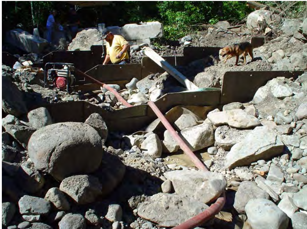
Photo A-8. The four weir plates prior to final backfill with angular material from the talus slope. The rise of the plates is clearly visible as is the offset of each one.
