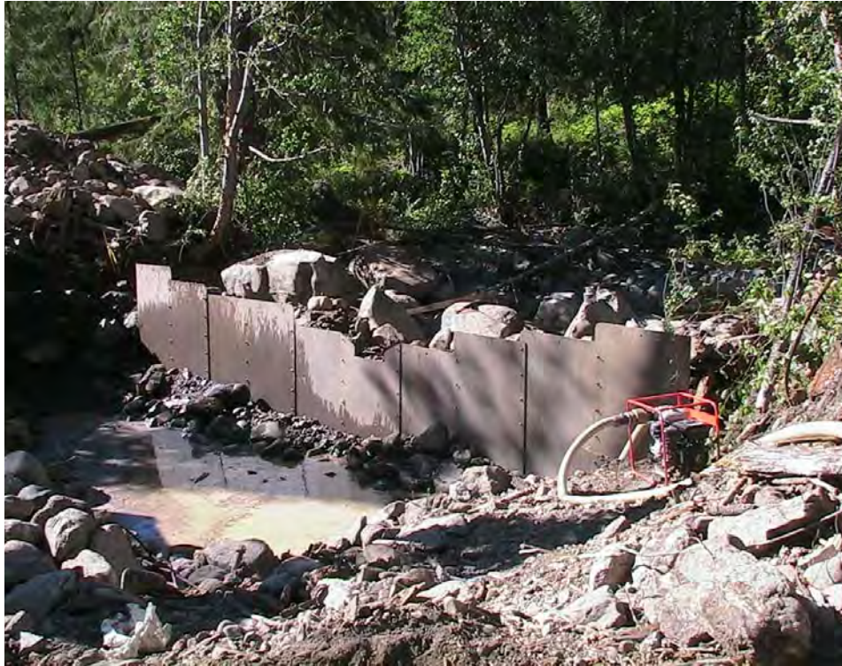
Photo A-7. A downstream view of Weir #4 prior to backfill. The bolted plate is almost completely buried in the existing streambed and should be nearly impossible to move. About 250 cfs can flow between the plates before the creek rises high enough to reach the banks above the plates. Channel capacity should be 700 to 900 cfs.
