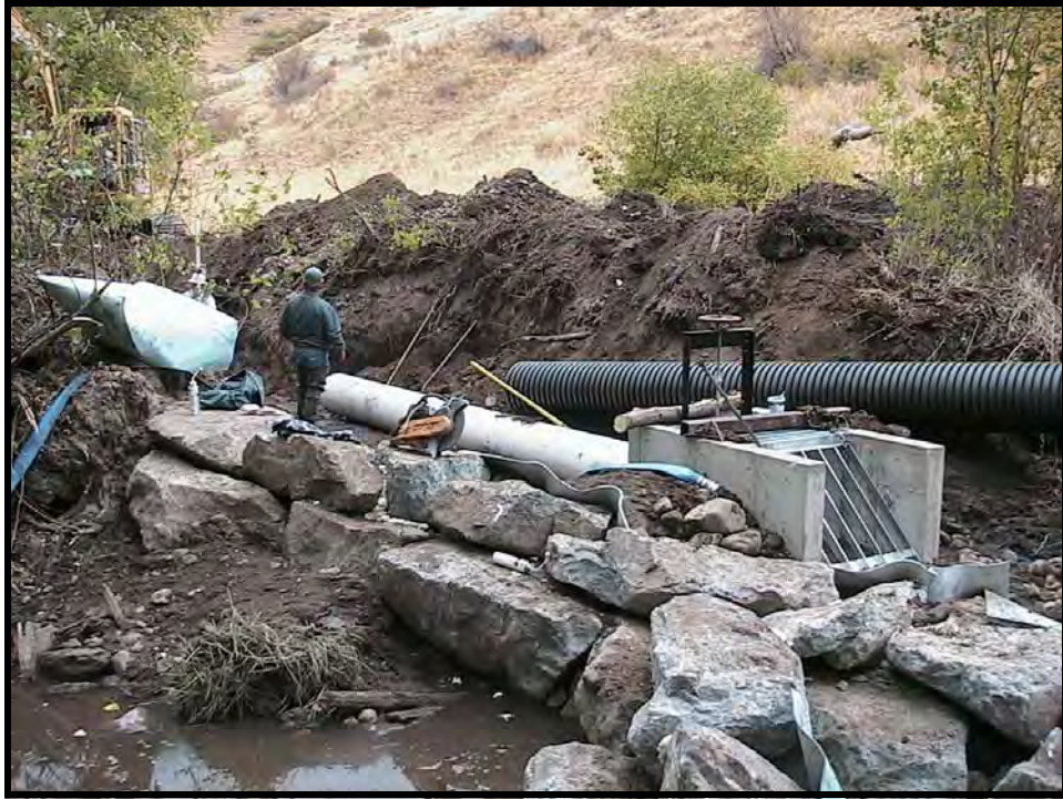
Photo A-10. Looking upstream across the right arm of Weir No. 1. The white PVC pipe is attached to the box's "stub." In a field modification to extend the irrigation further down the ditch, the corrugated black HDPE pipe was attached to the PVC pipe.
