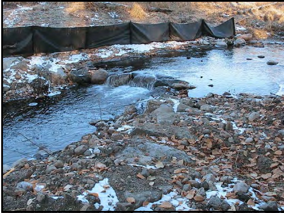
Photo A-19. Weir No. 2 during low flow on November 15, 2003. The silt fence in the background will remain in place until the spring of 2004.
