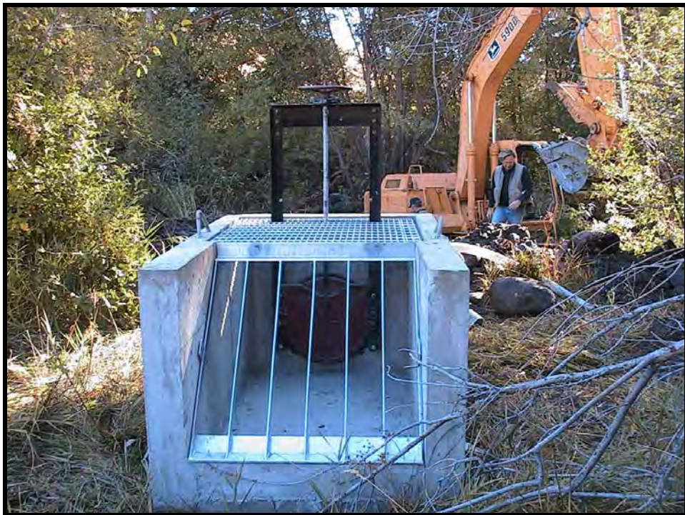
Photo A-8. The intake side of the new diversion box, before placement. Both the trashrack and the grate(on top) are galvanized.
