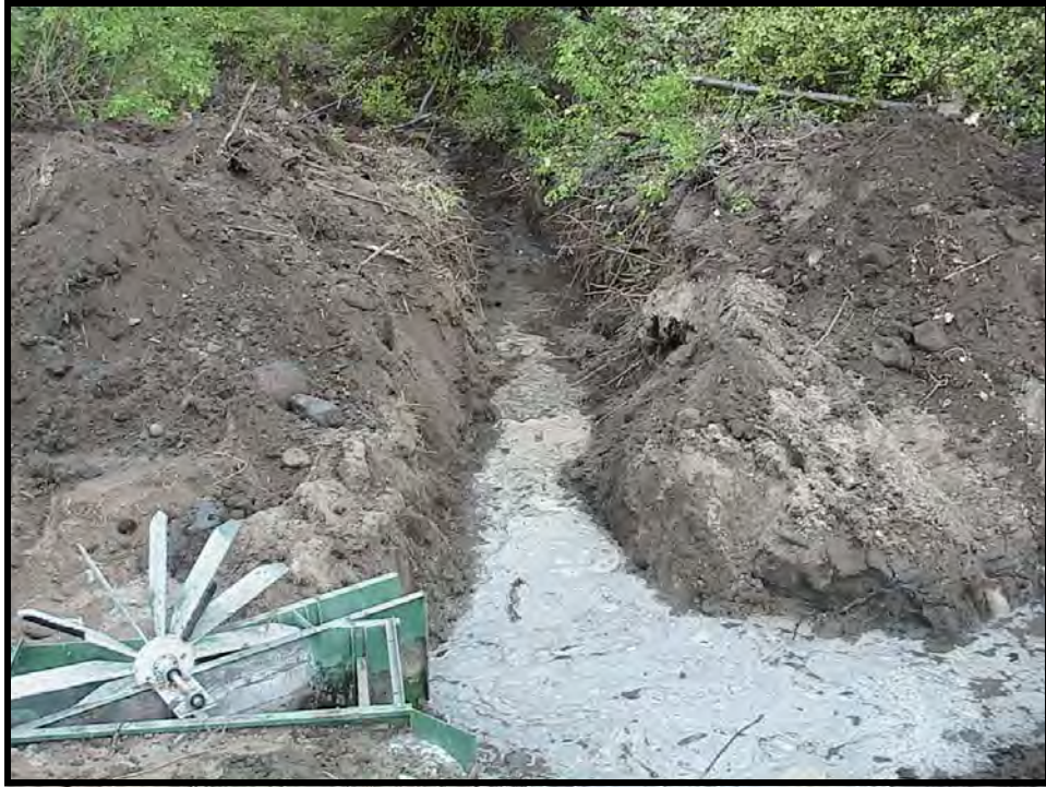
Photo A-15. The fish bypass channel, before installation of the fish bypass return pipe.
