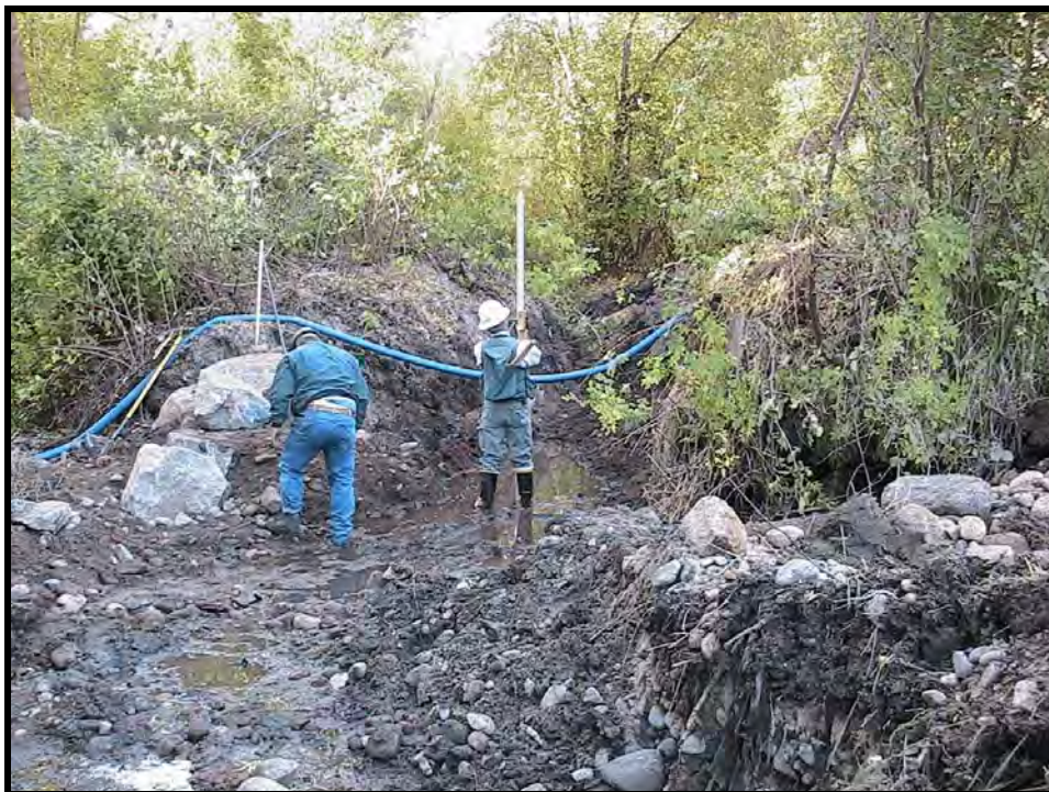
Photo A-4. Looking downstream at site of Weir No. 1 as technicians set elevation for the new diversion structure. The existing ditch was excavated about 12 inches to serve the lower elevation of the new headgate.
