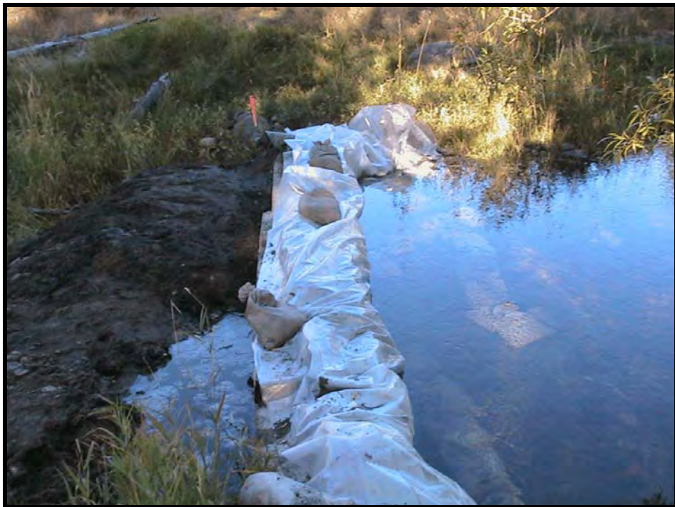
Photo A-2. The ecology block and plastic cofferdam was set about 80 feet upstream from the original diversion dam.
