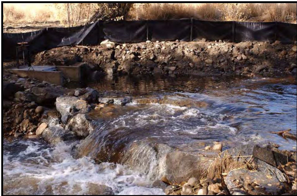
Photo A-24. November high flow over the double-drop Weir No. 1, which is the diversion control structure.
