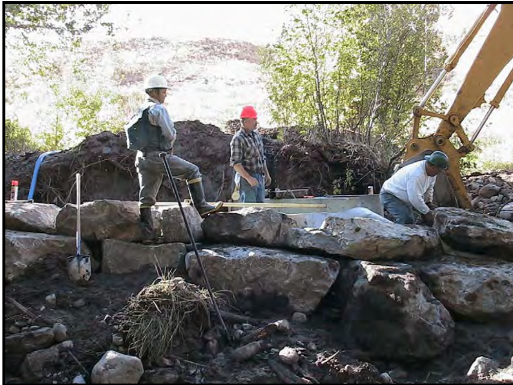
Photo A-5. Looking upstream at the left arm of Weir No. 1. Diversion structure is set in the center of the photo. The large rocks were brought in from a quarry about 30 miles east. Note the even slope of the rocks and lack of gaps between them.
