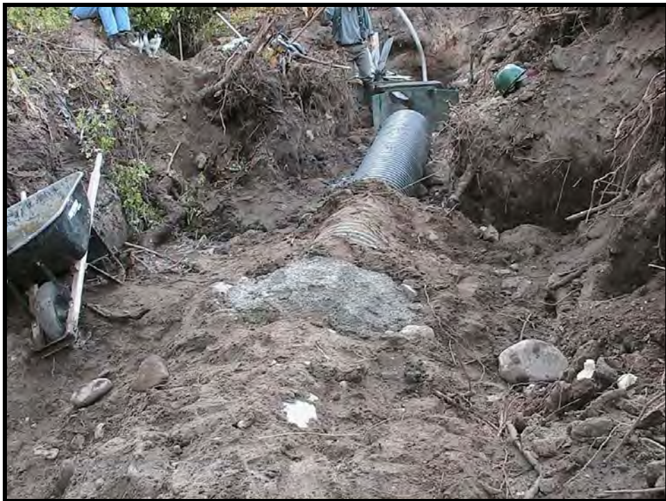
Photo A-12. The concrete protects and weights the transition between the PVC (white) and HDPE (black) irrigation pipes (see photo A-10). The fish screen is in the upper center of the photo, just above the black pipe.
