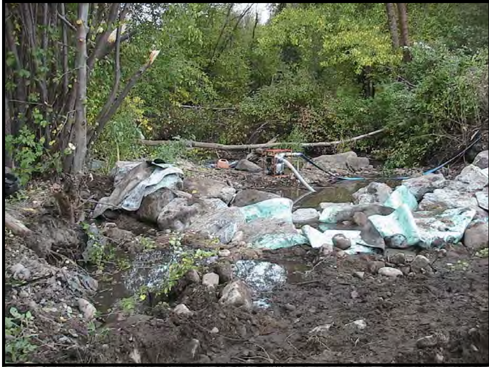
Photo A-7. Downstream view of Weir No. 1; the non-permeable geomembrane has been installed but not fully covered.
