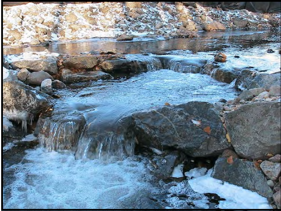
Photo A-23. At Weir No. 1, the drop at the downstream portion is greater than designed. After highwater in 2004, if the bed of the pool has not been built up by deposited gravels, the drop will be adjusted.
