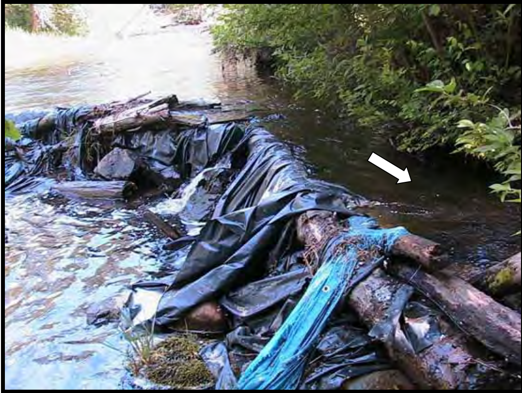
Photo A-1. Looking upstream at original Thurlow Transfer Ditch diversion dam. The ditch is on left side of Beaver Creek, between the Upper Stokes and Lower Stokes diversions. Arrow shows direction of flow of ditch water.
