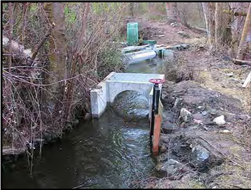
Photo A-30. Looking up the Thurlow Transfer Ditch. The headgate to the new 12-inch sluiceway is in front and the fish screen in the background. (April 2004)
