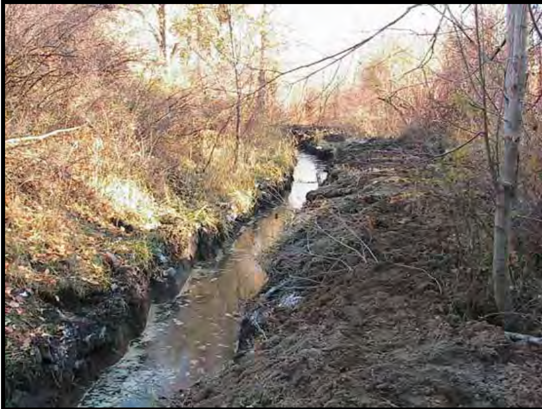
Photo A-22. View from fishscreen looking down diversion ditch.
