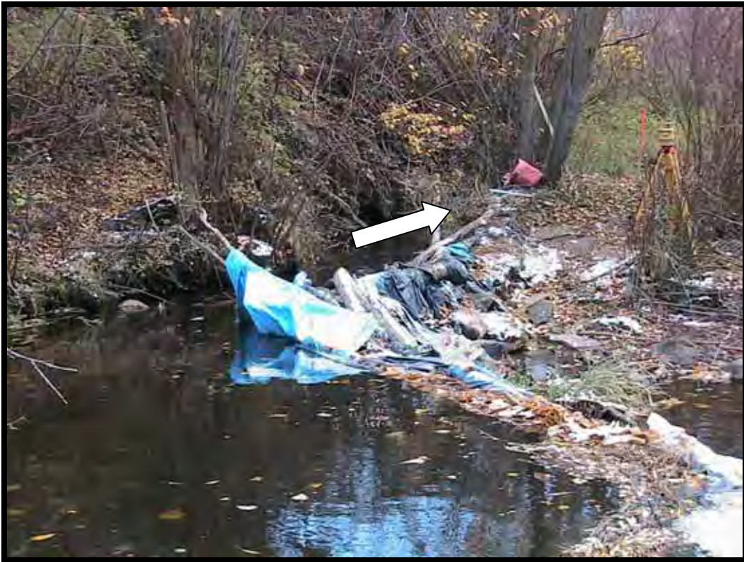
Photo A-5. Looking downstream at the original diversion dam; the arrow shows the direction of flow of the ditch.
