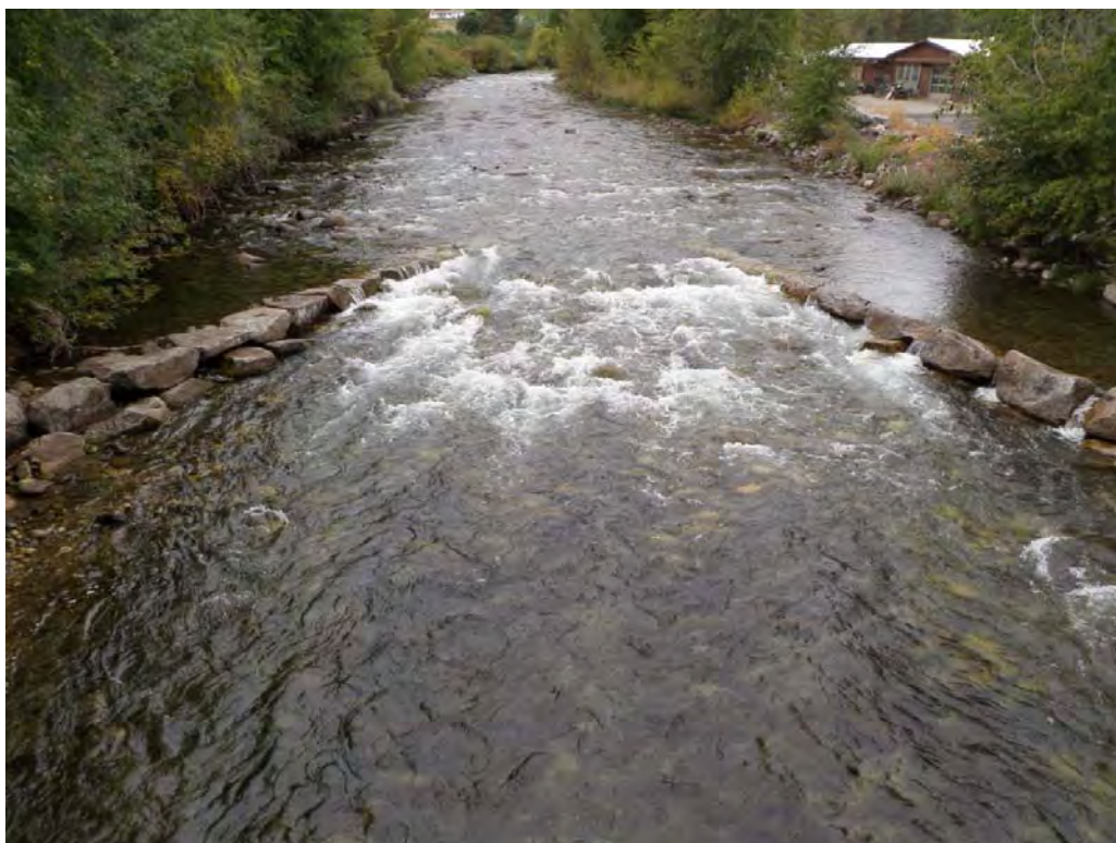
Figure 18. Dinkleman cross vane structure in the Entiat River at RM 4.6 in 2011, roughly 10 years after construction and one 10-year flood. As opposed to creating a scour pool as anticipated, most of the area near the apex of the weir has filled in with coarse bedload.
