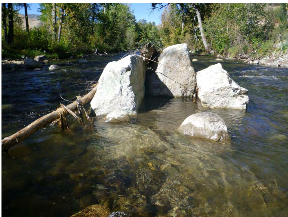
Figure 39. Constructed boulder cluster in the lower Entiat River near RM 1.4.
