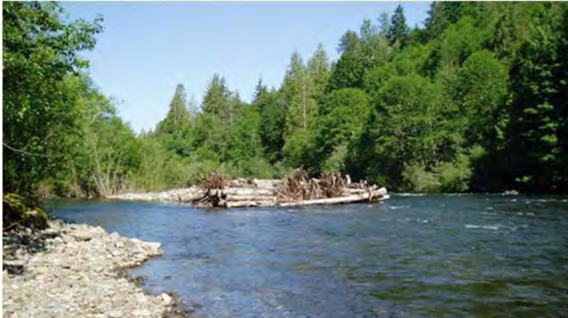
Figure 37. Constructed mid-channel ELJ located on the Green River, Washington (courtesy Anchor QEA).
