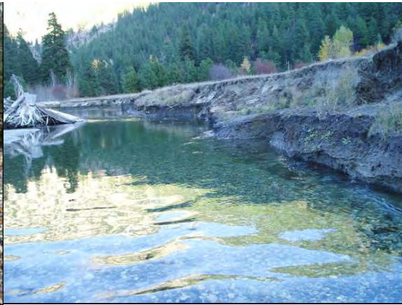
Eroding bank at RM 21.4
