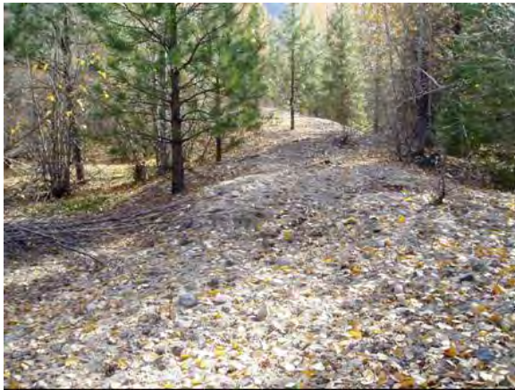
Dike above left bank at RM 22.4
