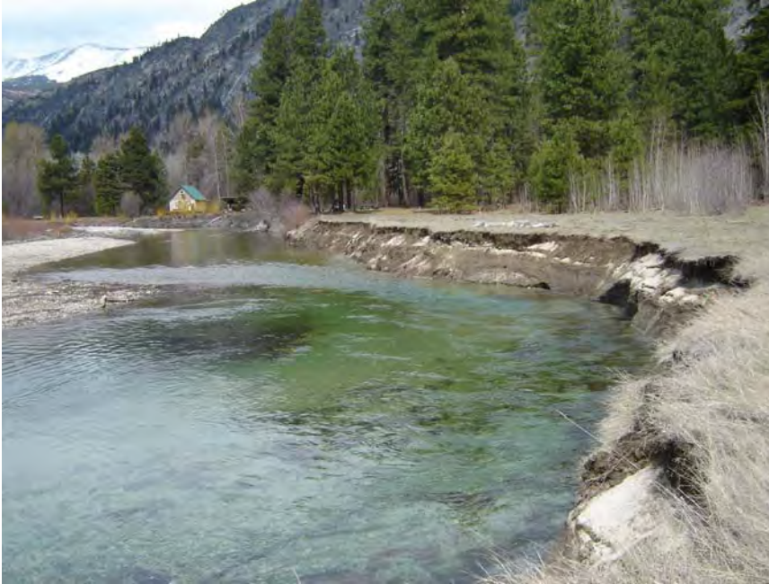
Figure 34. Bank instability at RM 21.5 (looking upstream).
