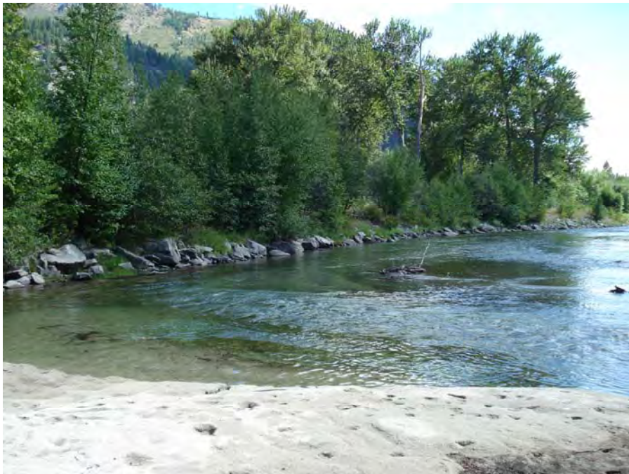
Photograph No. 42. View is to the south looking at riprap placed along a levee on river left. Preston Reach – Entiat Subbasin, Washington – Bureau of Reclamation Photograph by R. McAfee August 21, 2008
