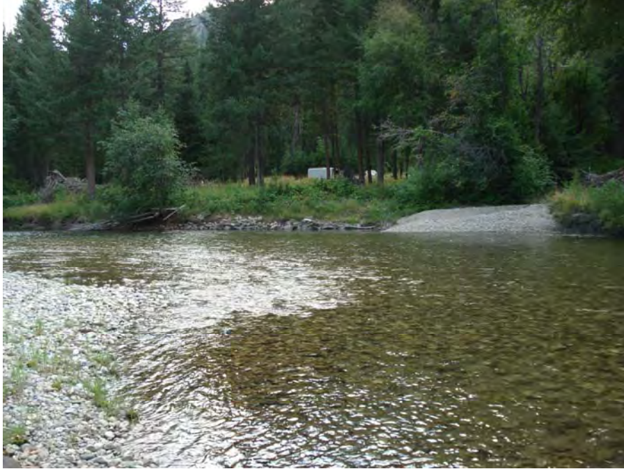
Photograph No. 37. View is to the southwest looking downstream where a tributary enters the Entiat River along river right. Note the gravel embankments (“training dikes”) placed along both streambanks of the tributary. Preston Reach – Entiat Subbasin, Washington – Bureau of Reclamation Photograph by R. McAfee August 21, 2008.
