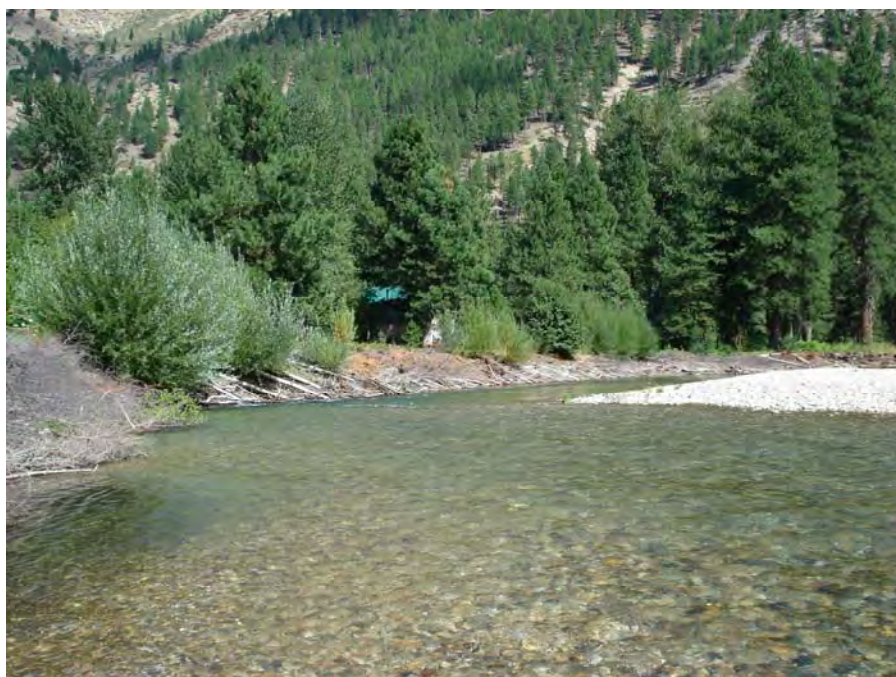
Photograph No. 32. View is to the east looking downstream at small-to-medium size wood being utilized for bank protection (“Christmas Tree Revetment”) along river left. Preston Reach – Entiat Subbasin, Washington – Bureau of Reclamation Photograph by R. McAfee August 21, 2008.
