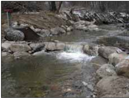
Marracci Weir After
