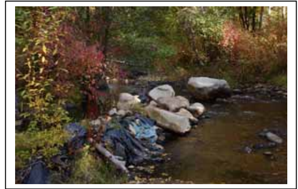
Marracci Weir Before
