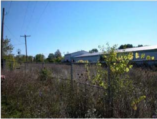
Eastern end, north facing side of the former Zonolite Co./W.R. Grace vermiculite processing building.
