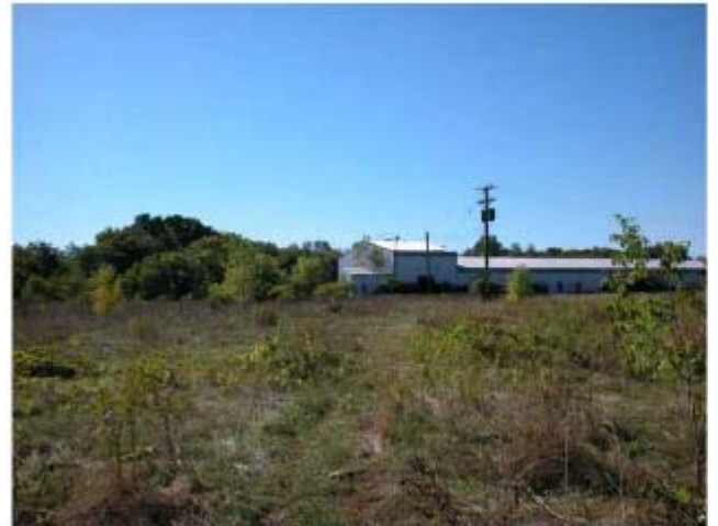
East end of former Zonolite Co./W.R. Grace vermiculite processing building. The storage silos were located immediately east of this building.
