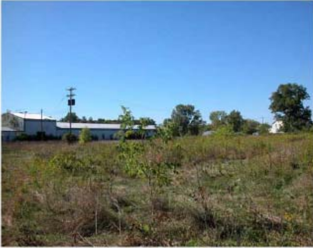
North facing side of former processing building.
