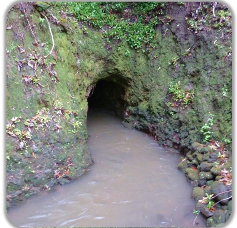
Manuel Luis Ditch, typical tunnel
