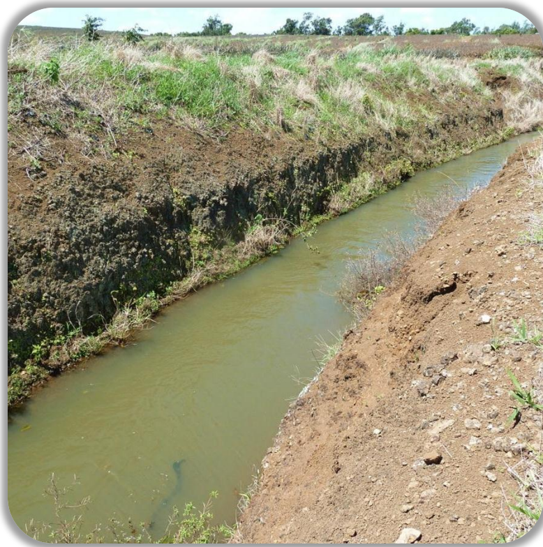
Lowrie Ditch, earthen walls and bottom
