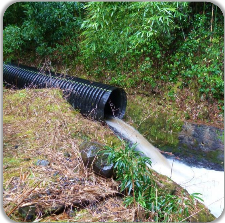
Lowrie Ditch, pipe section of the ditch
