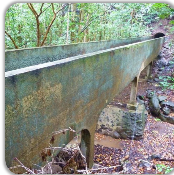
Haiku Ditch, concrete flume
