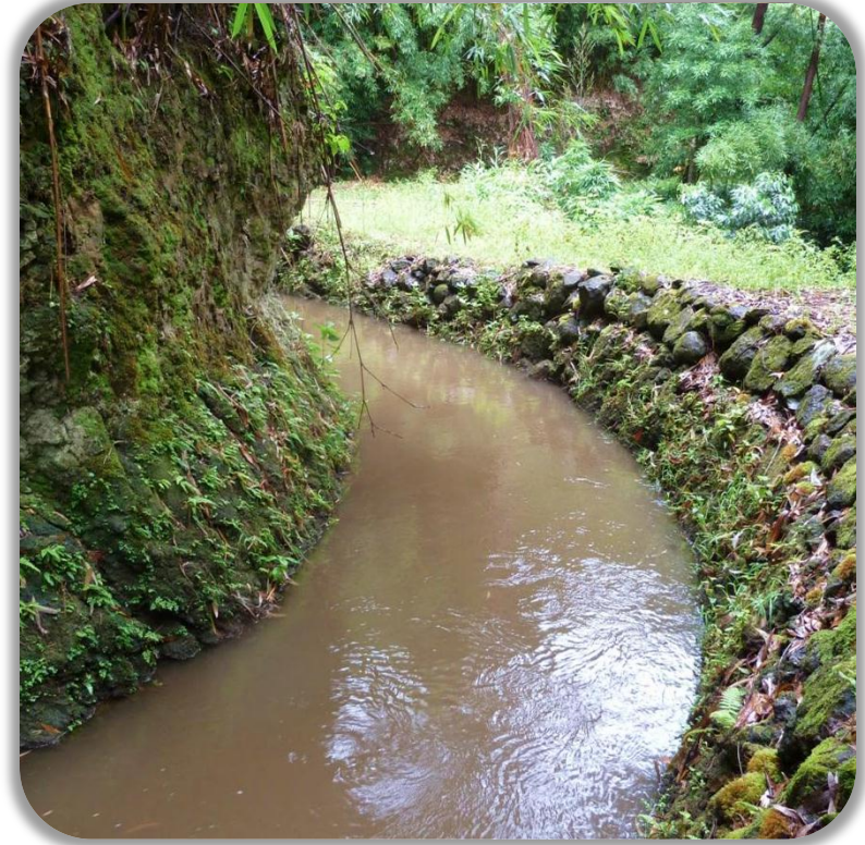
Center Ditch, stacked rocks on right wall and bedrock on left wall
