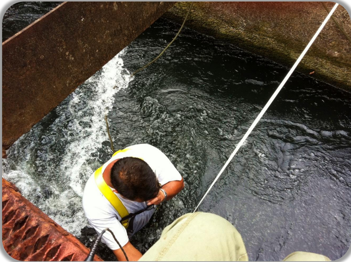
Wailoa Ditch at Halehaku Flume
