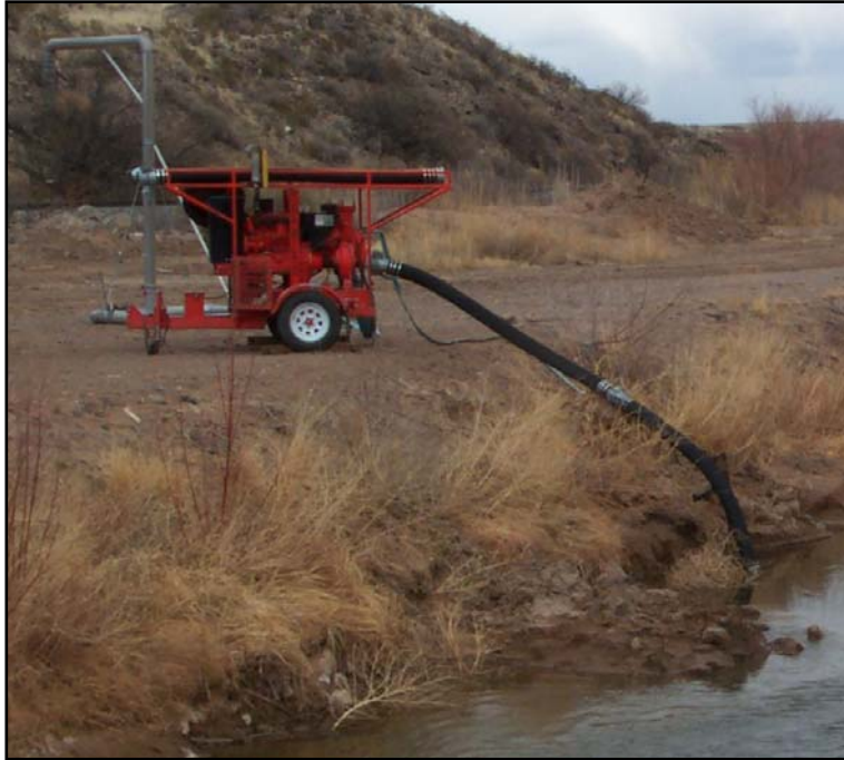
Figure 2. Typical water pump setup for dust abatement.
