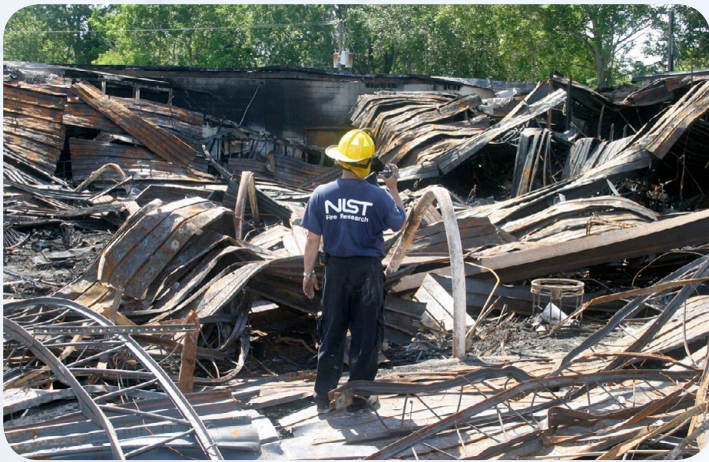
NIST researcher photographing the remains of the Sofa Super Store in Charleston, S.C., on June 19, 2007, the day after the fire that killed nine firefighters.
