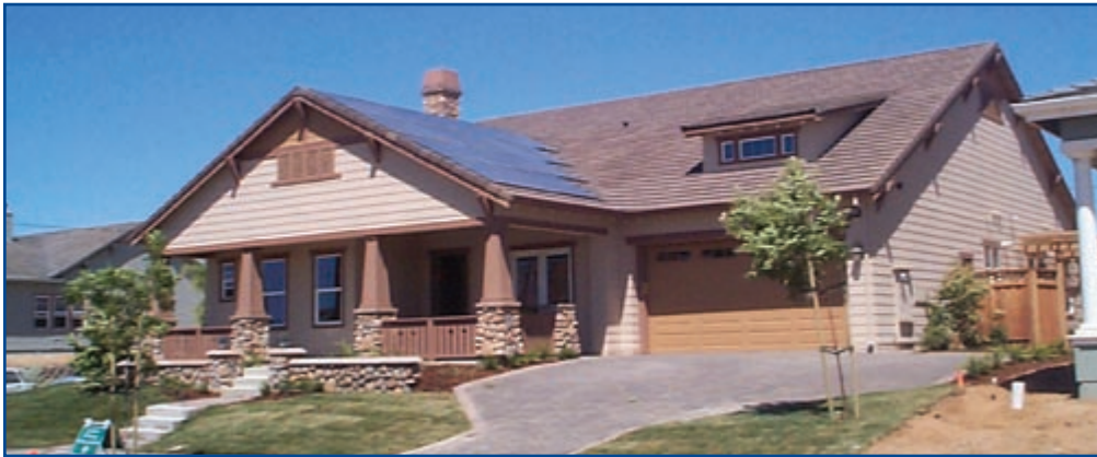
Southwest view of the Centex 21st Century Performance Home in Livermore shows 3.6-kW photovoltaic panels on the south-facing roof.
