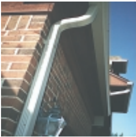
Gutters and downspouts
