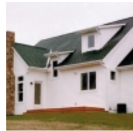
Proper grading around house
