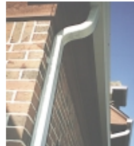
Gutters and downspouts
