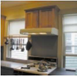
Kitchen exhaust hood
