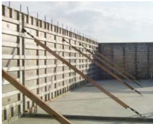
Figure II-17. Prefabricated aluminum forms in place and braced
