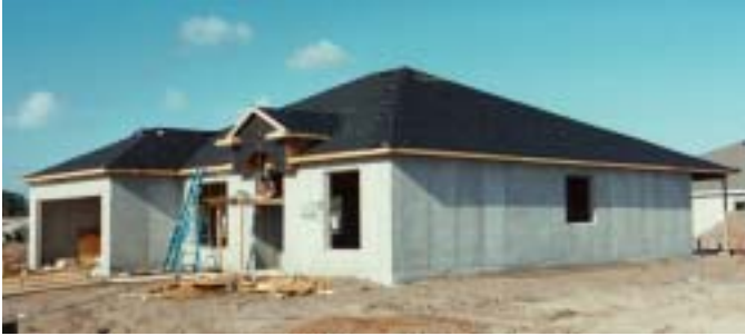
Figure II-29. Mercedes Homes fourth prototype under construction
