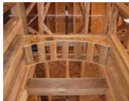
Figure III-14. Framing box-downs are not air-sealed
