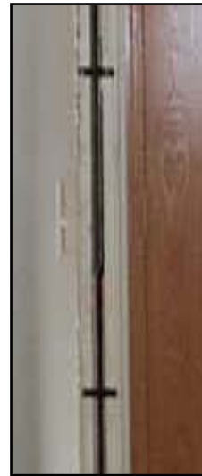
Figure I-44. Gasket seal at marriage wall
