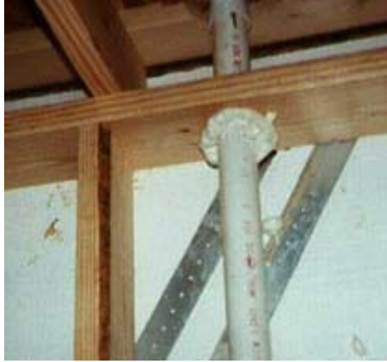
Figure I-5. Sealing techniques
